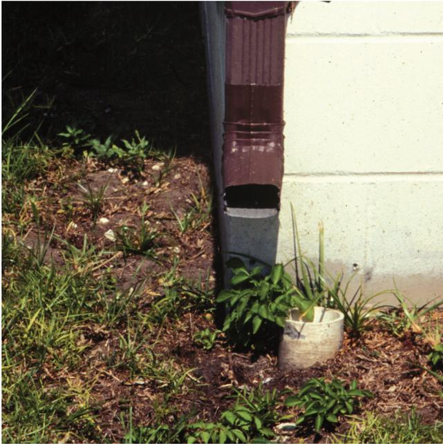
Short down spout causes improper drainage at foundation.
